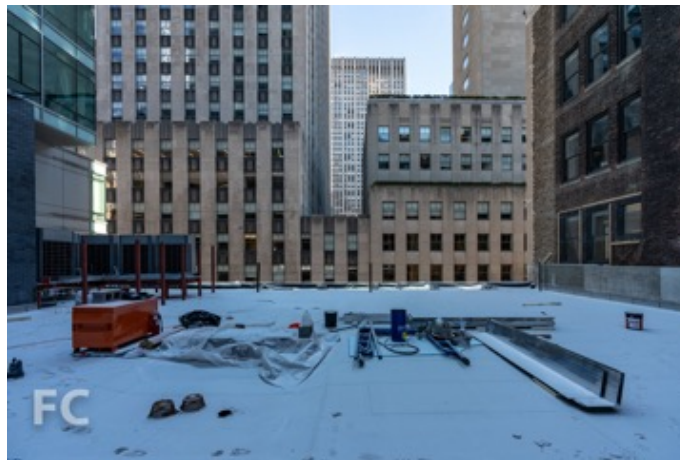
Future rooftop terrace at the fifth floor.
